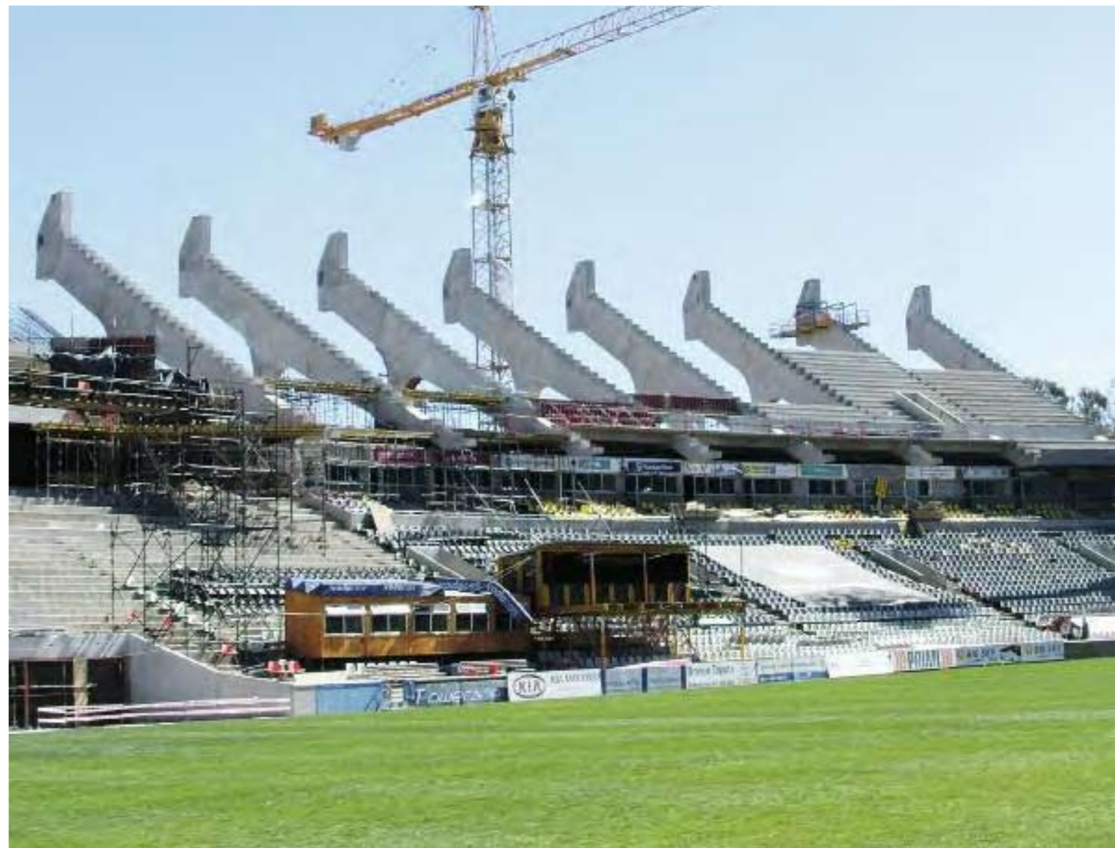
© Médiathèque Lafarge – Elso Consulting Engineers
